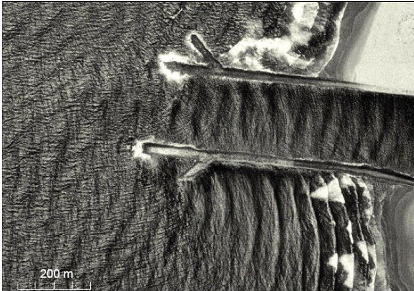
Example of jetty spurs at Siuslaw River Inlet, OR. Spur lengths are 122 m
